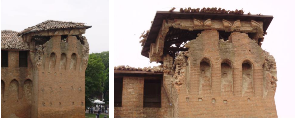
Fig.1 San Felice sul Panaro fortresses: effect of seismic action on merlons reinforced with excessively rigid ribs.
