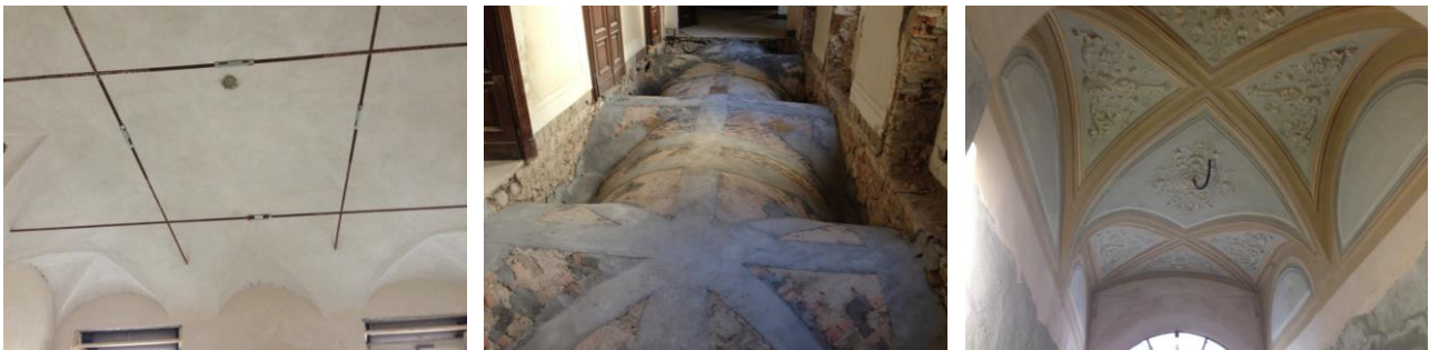
Fig.3 Masonry vaults reinforcement: (a) insertion of tie-rods; (b) FRCM-PBO system applied at the extrados; (c) Frescos at the intrados of cross-vault.
